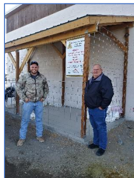
Chemical container recycling bin
