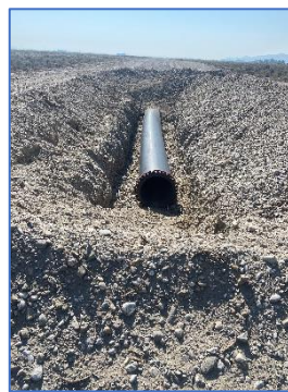
NRCS funded irrigation ditch to pipeline conversion project
