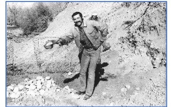
Walt Johnson building rock gabions for a conservation project in 1980
