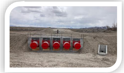
Fish Screens Installed in the Little Lost River Valley
