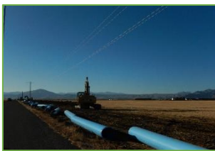
Pipeline project, Butte County
